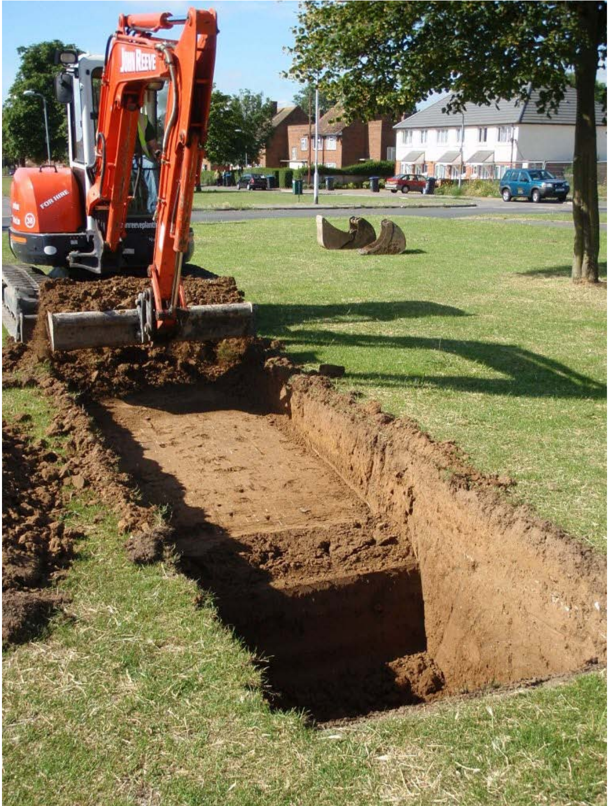
Plate 1 Test Pit 1 Working Shot looking South West – 1m scale
